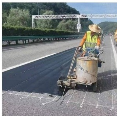
reticular crack
