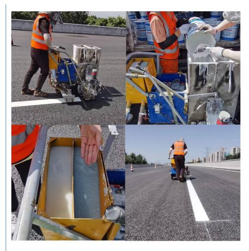
HG-20MM-II puts two kinds of coatings in the same barrel separated. After discharging the coatings from the tank, the coatings are fully stirred by an electric stirring shaft. After mixing in the crossing hopper, the chemical reaction is carried out. Finally, the marking is done through the crossing hopper. Compared with spraying two-component marking, scraping marking has the advantages of:
