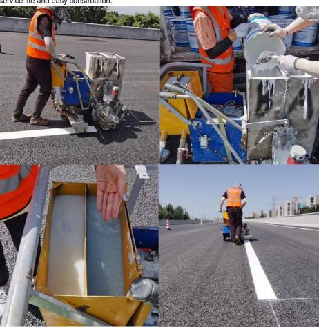
HG-20MM-II is to put two kinds of coatings in the same barrel separated. After discharging the coatings from the tank, the coatings are fully stirred by an electric stirring shaft. After mixing in the crossing hopper, the chemical reaction is carried out. Finally, the marking is done through the crossing hopper. Compared with spraying two-component marking, scraping marking has the advantages of thicker marking thickness, longer wear resistance, better reflectivity and more uniform mixing.
