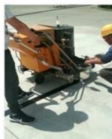
Thermoplastic road marking machine
