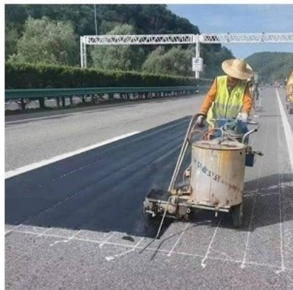
reticular crack
